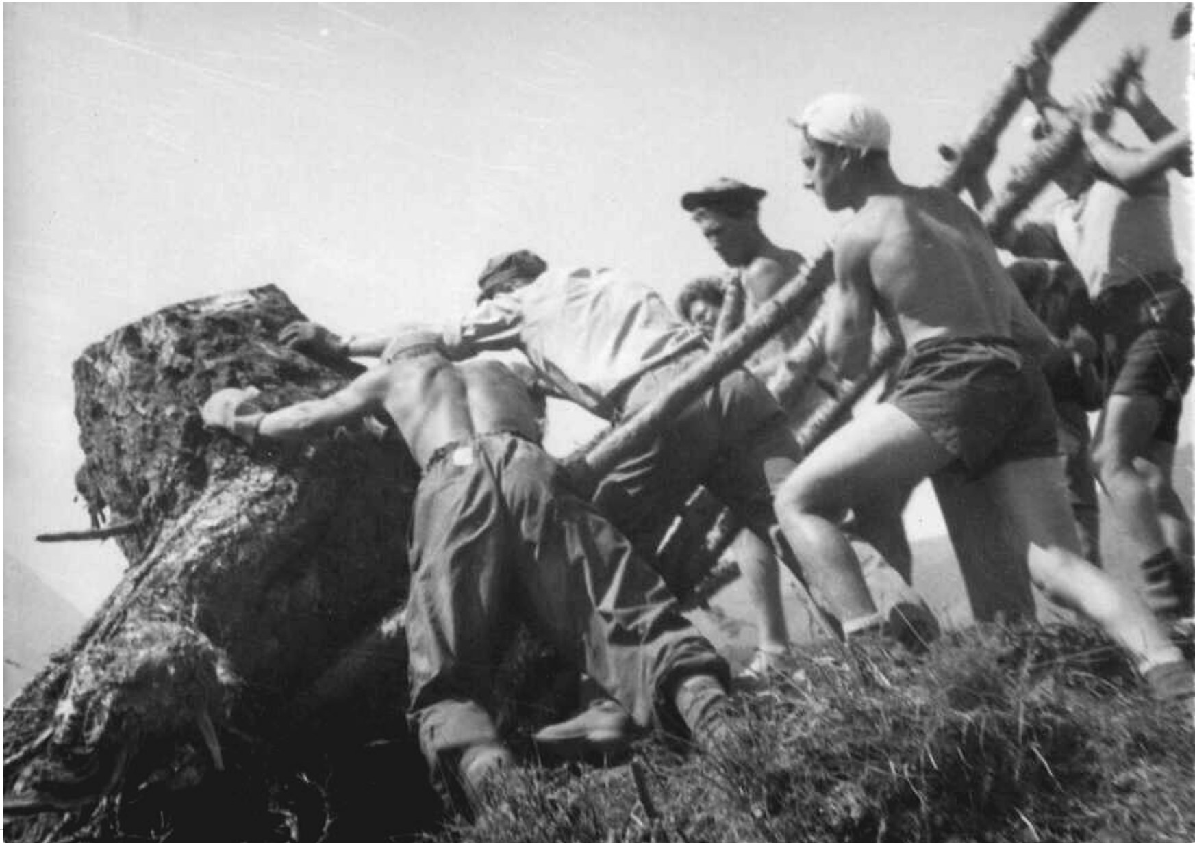
No.13 Feldis (Switzerland) Hard cleaning work after flood
